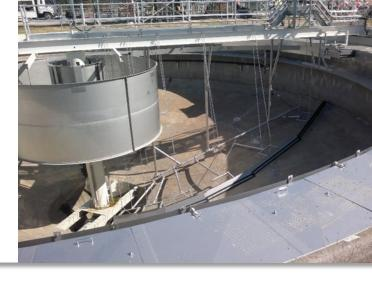
In operation since in the 1970's, the original clarifiers were removed and whilst some parts were retained, the new internal equipment provided by EPCO Australia was designed to suit the geometry of the existing clarifier tanks.
